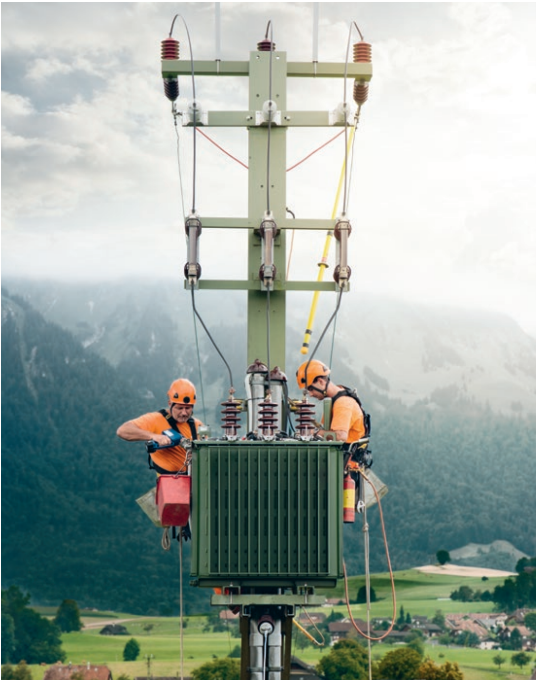
Smart technology allows traditional local grid transformers to regulate problematic voltage differences directly in the network, as seen in the photograph.
