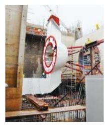
Hagneck hydroelectric power plant: installation of a turbine housing in December 2013.
