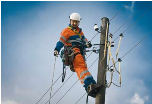
→ Grid technician at work
