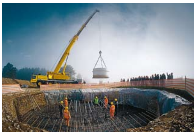
→ Construction work on Mont-Crosin wind farm
