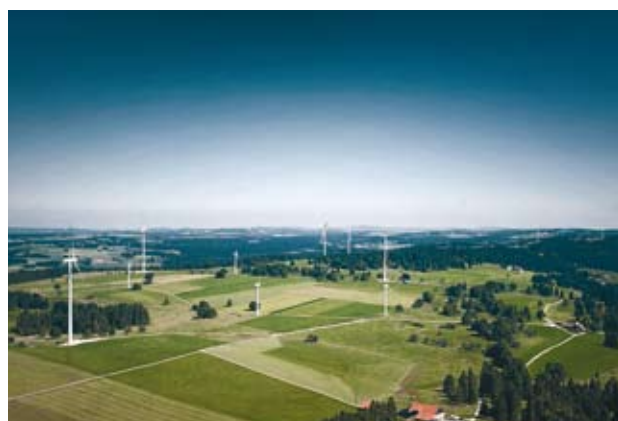
→ Switzerland's biggest wind farm on Mont-Crosin
