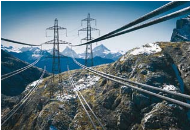
→ Ultra-high-voltage grid in Gemmi Pass
